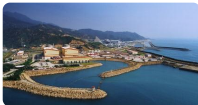
first large commercial nuclear power station in mainland China
